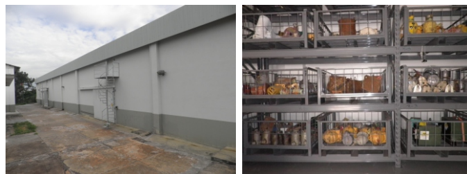
Figure 4. New radioactive waste storage building (outside and inside view).
